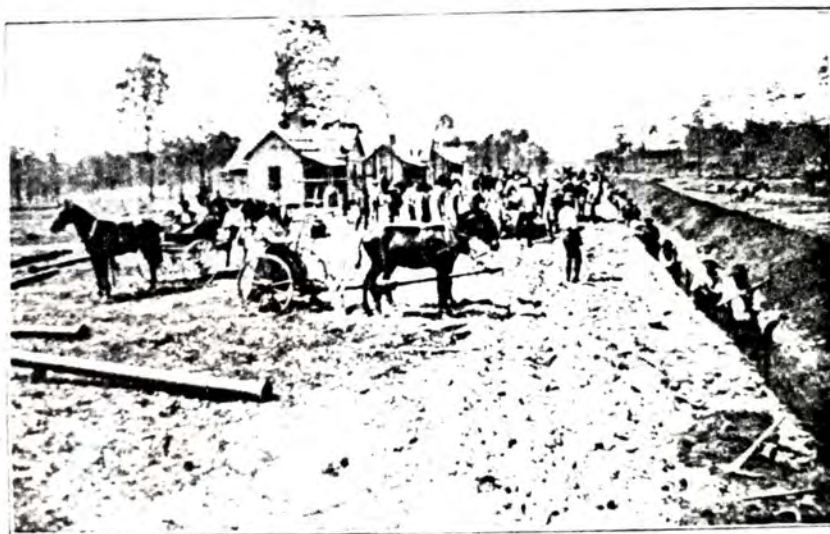
Figure 10. Morelia Avenue, May, 1902: "Showing the grading of the street and the laying of the eight inch water main."
